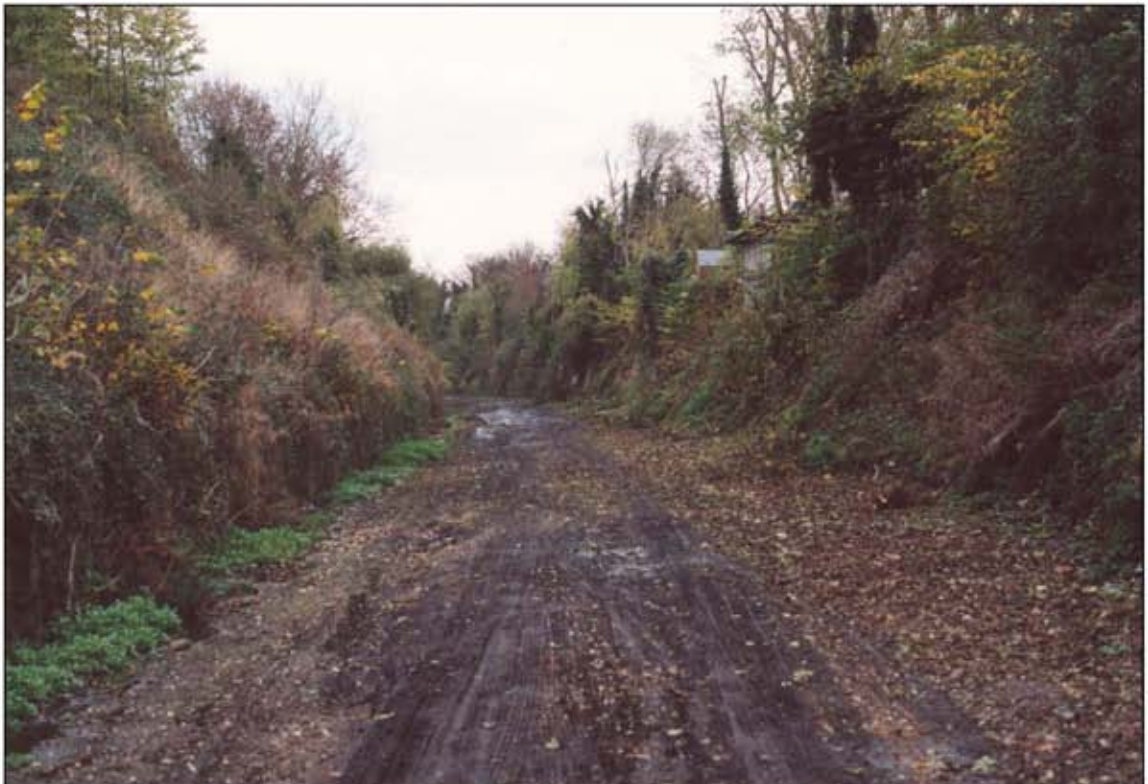
Plate 2 Railway cutting at Balally, prior to works taking place
