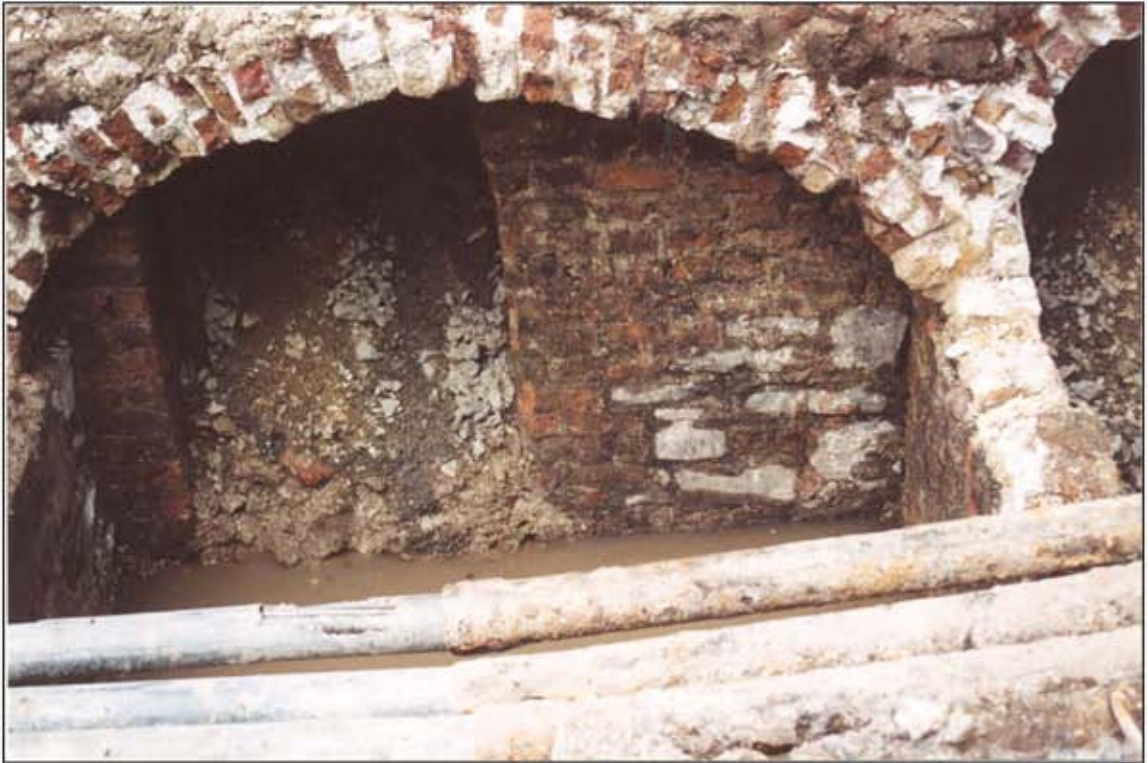
Plate 1 Exposed coal cellar at Harcourt Street
