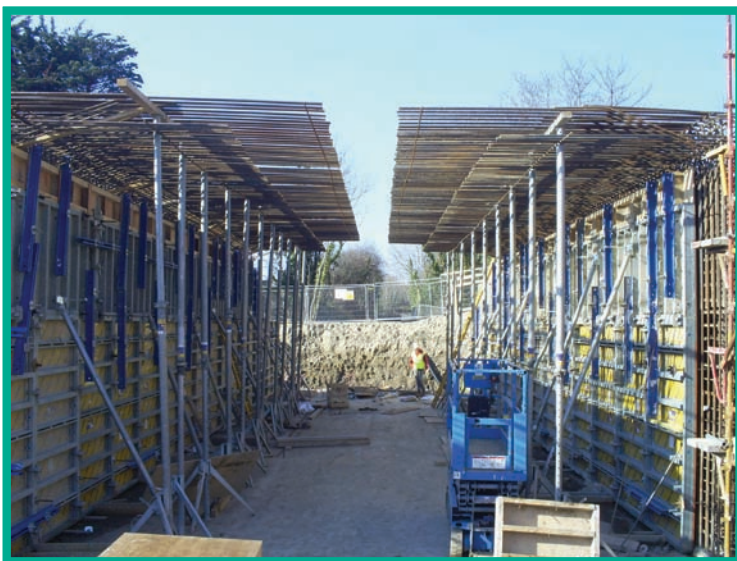
Formwork for wall pours on Glenamuck Bridge
