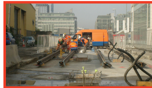
Track Works near The Point
