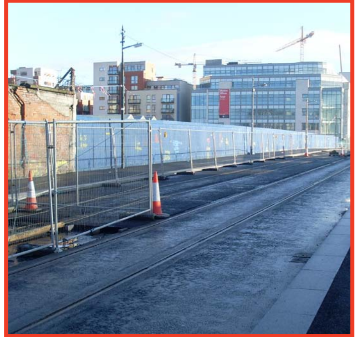
Mayor Street Upper finished track
