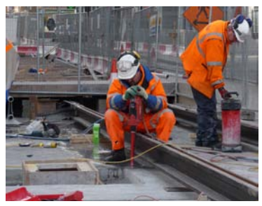
Track Works on Mayor Streer Lower
