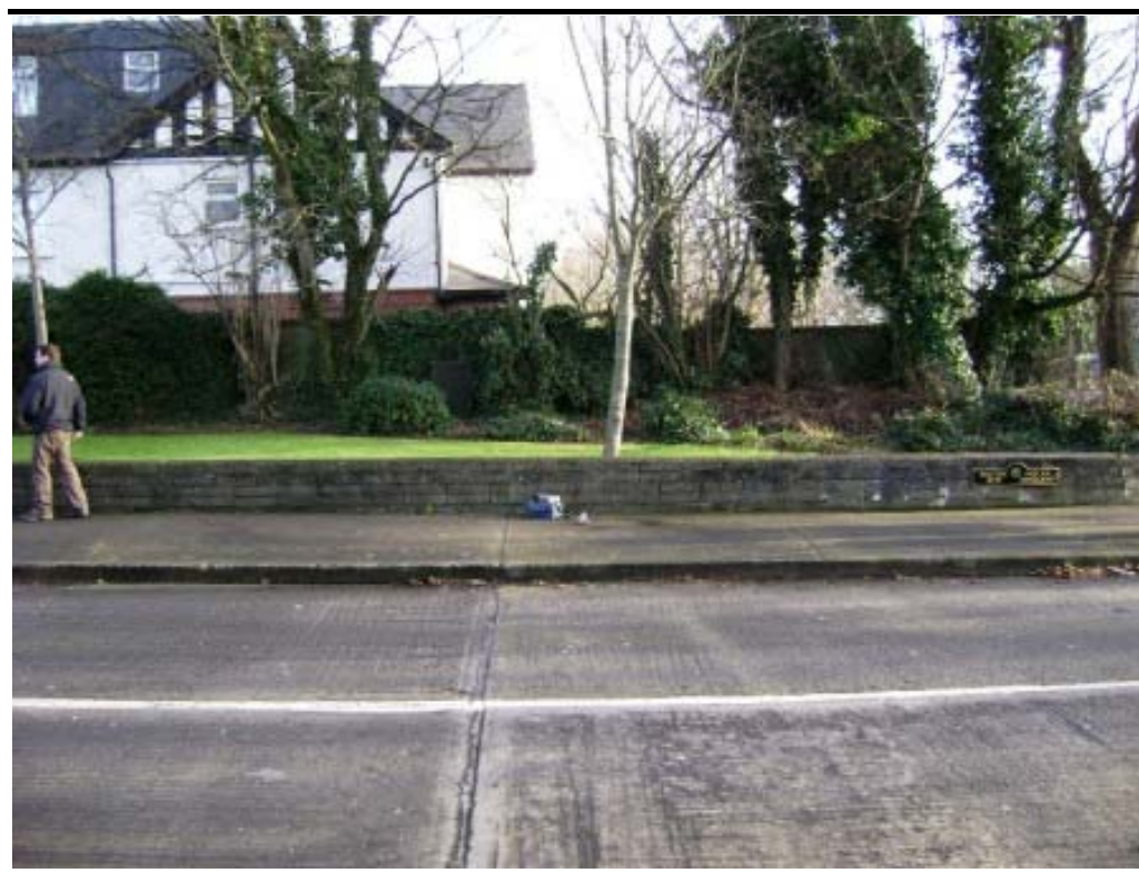
Figure A1.2 Griffith Ave / Walnut Rise
