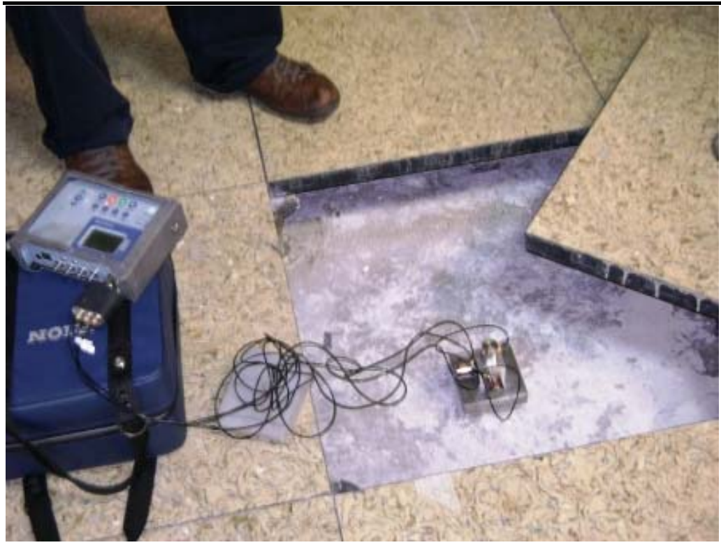
Figure A 1.7 Mater Private: Concrete floor in room adjacent to MRI machine
