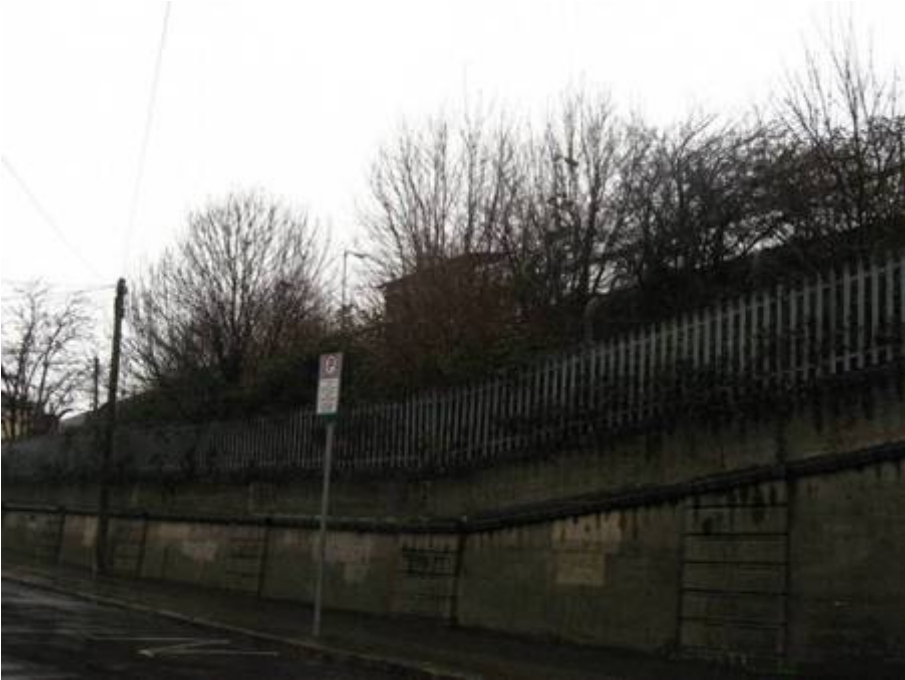
Figure 7-1 Retained embankment (looking at south side) carrying twin railway tracks
