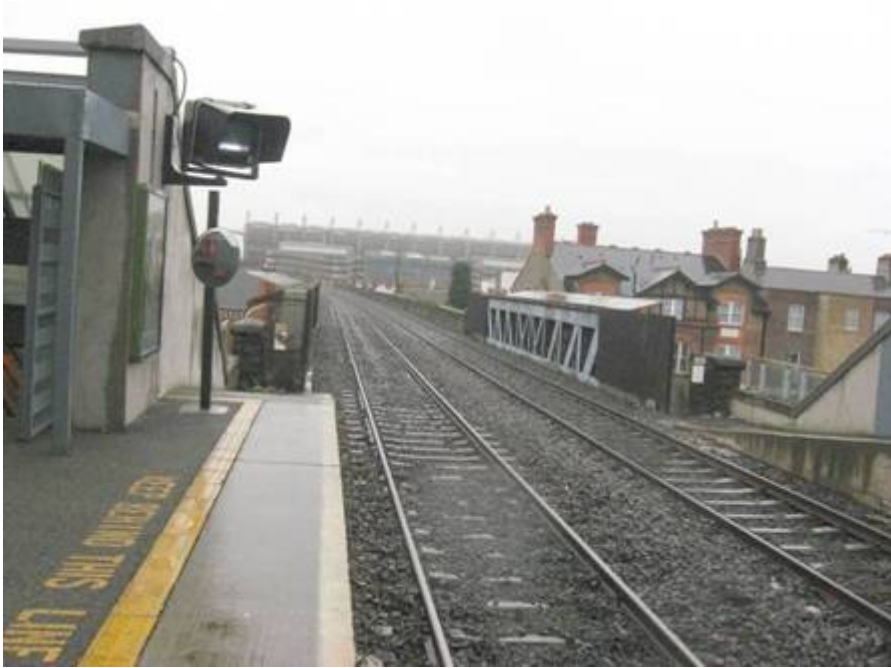
Figure 7-2 Twin railways tracks running along top of retained embankment
