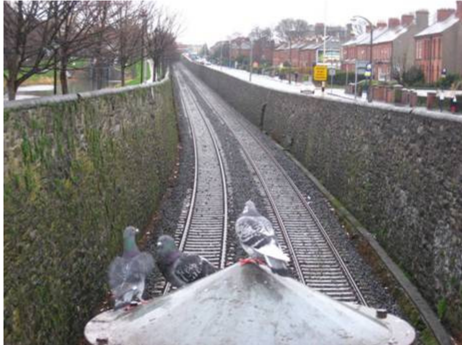
Figure 7-3 Twin Track Railway Line in Retained Cutting
