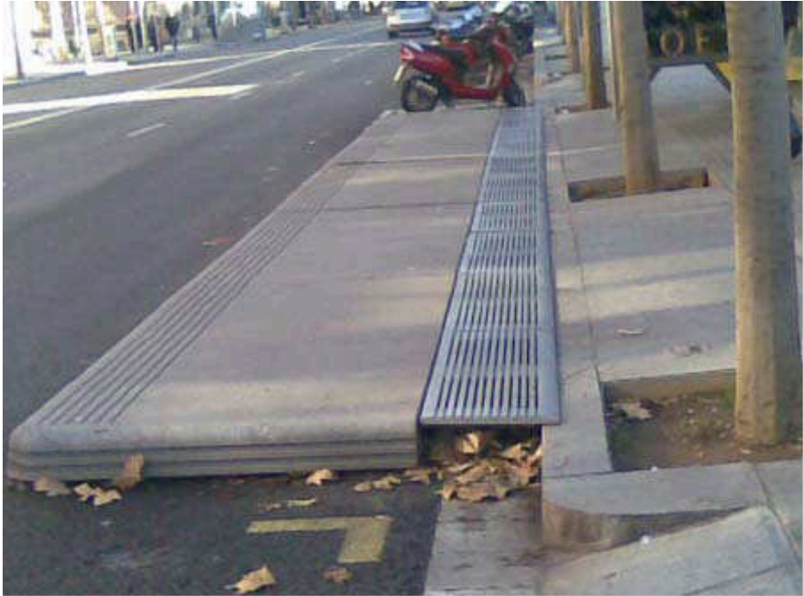
Figure D.1 Examples of Temporary Footpath Extensions
